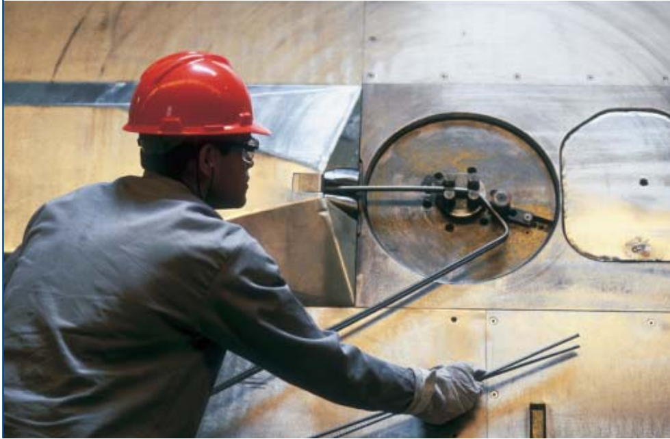
Rebar fabricating service
